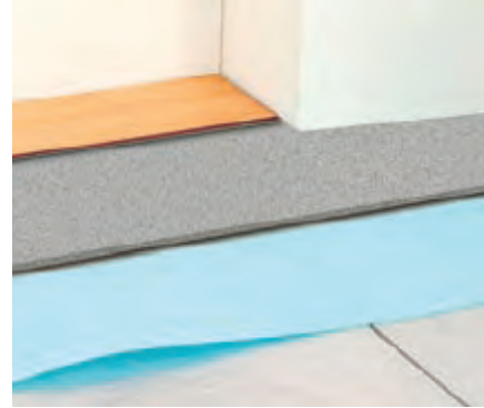
Fig. 13: Fitting of final floor structure
