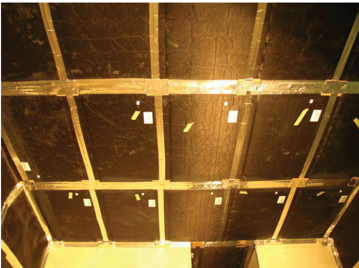
Figure 5: Standards sized 40 mm VIPs were used for internal insulation of the SELF unit. All joints are sealed with vapor barrier tape.
