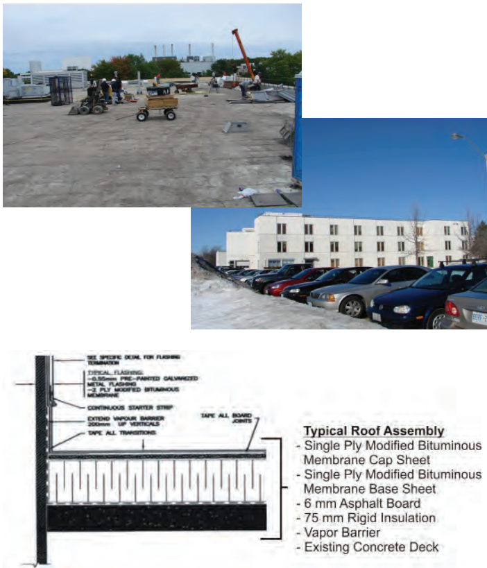
Figure 5: Re-Roofing of Building M-24 at NRC with Rigid Roofing System
