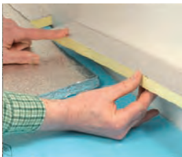
Fig. 11: Fitting of final PU-foam strip
