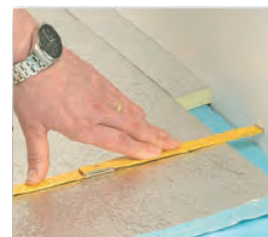
Fig. 8: Measurement of first circular "Cut"-layer
