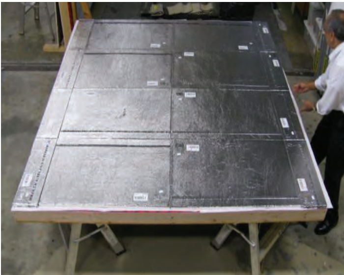
Figure 4: installation of the staggered second layer of VIP Type 2-Rounded edges
