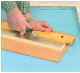
Fig. 9: Customizing of PU-foam strip
