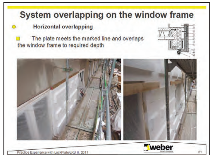
Figure 8. Window frame – horizontal overlapping
