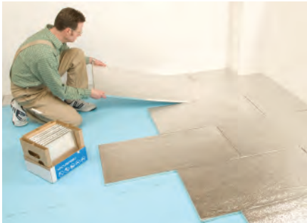
Fig. 10: Laying of modular VIPs
