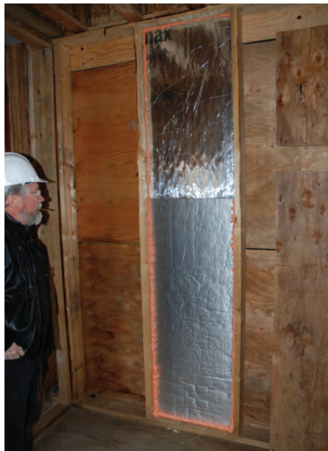
Figure 6: Harmony House initial exterior wall construction showing VIP in lower portion of wall with foil faced isocyanurate foam board behind.
