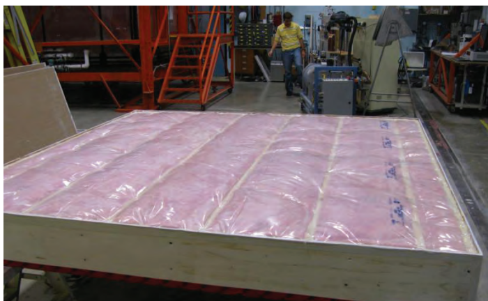
Figure 6: Polyethylene Air & Vapour Barrier sealed on perimeter
