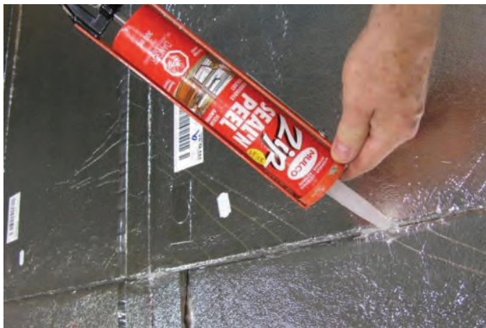
Figure 5: Sealing edges with silicone
