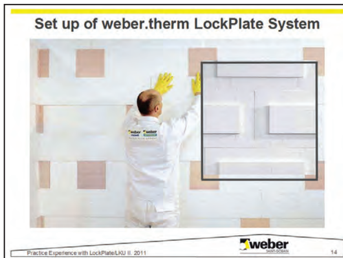
Figure 5. LockPlate set up
