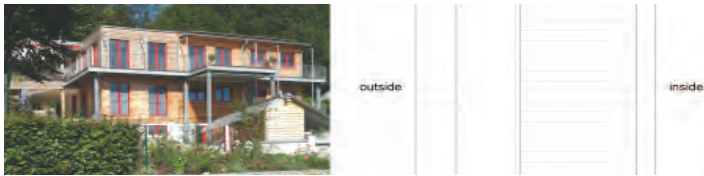
Figure 2: Case study 2: Single family house in Neumarkt (Germany), 2004. Design by Martin Forstner. Image by: Variotec.
