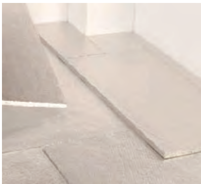
Fig. 12: Laying of second VIP-layer
