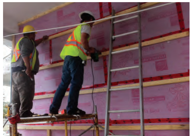
Fig. 7. Installation of the horizontal support members over the polystyrene layer.
