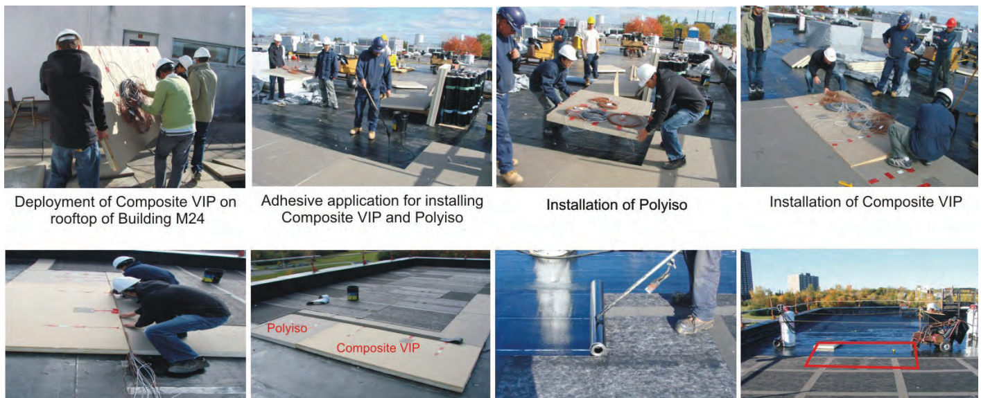
Figure 8: Installation Of Composite VIP And Polyiso On M-24 Roof System
