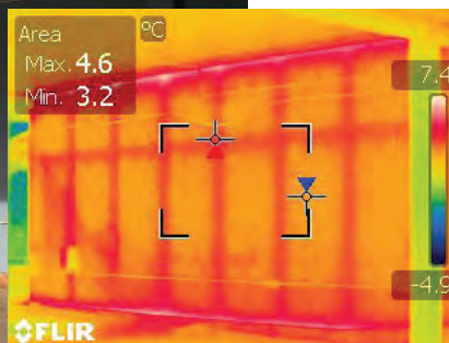
Fig. 5. Infrared Image of the wall selected for the VIP pilot.
