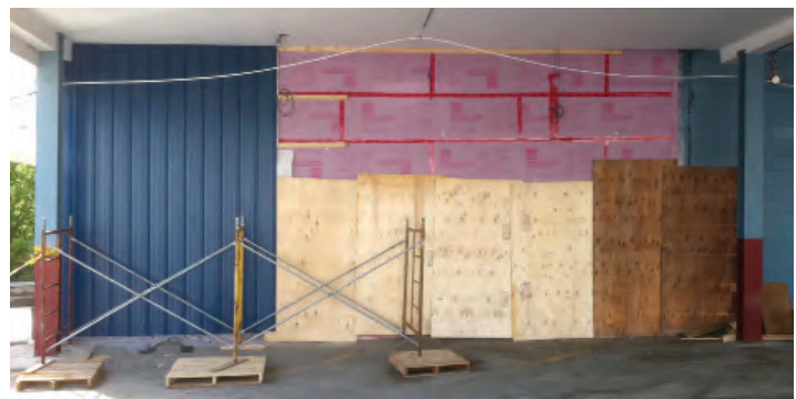
Fig. 10. Installation of the second layer of polystyrene. Plywood was used to cover unfinished work overnight.
