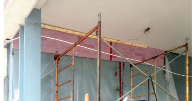
Fig. 6. Installation of the air/vapour/moisture barrier.
