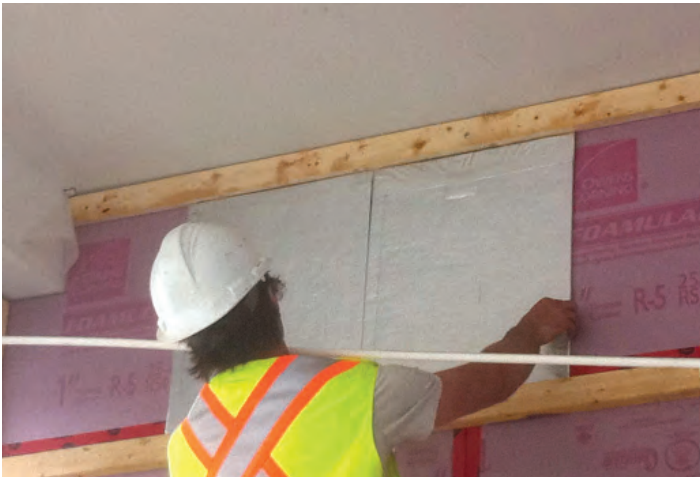
Fig. 8. Installation of the vacuum insulation panels (VIPs).
