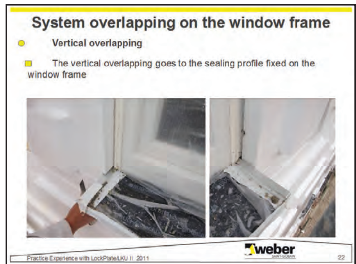
Figure 9. Window frame – vertical overlapping
