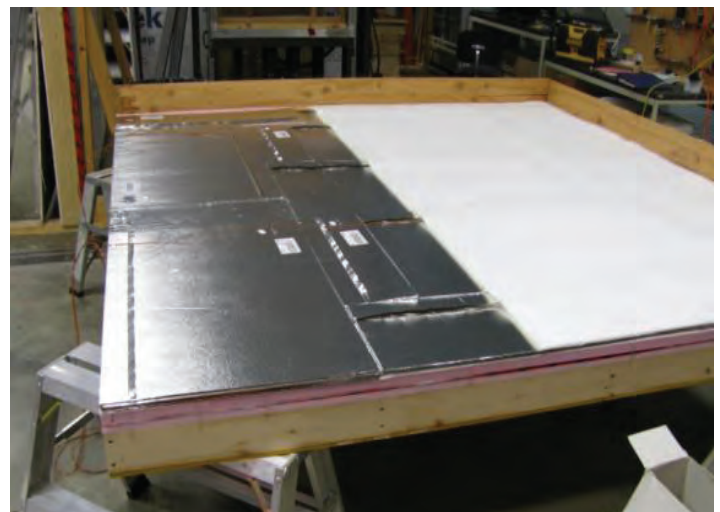
Figure 3: Installation of the first layer of VIP Type 2-rounded edges
