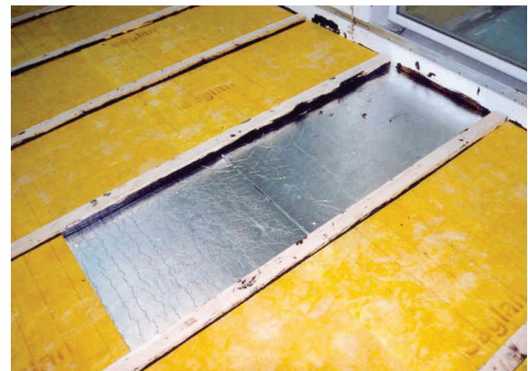
Picture 4: VIP protected by glass wool and by a timber panel. It can be replaced easily.
