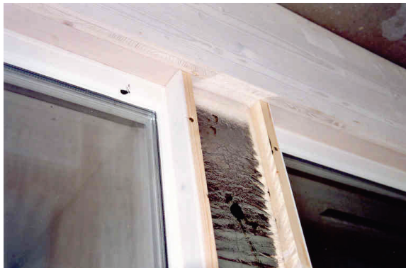
Picture 3: Window frames are covered with custom sized VIP. The VIP is protected by a wooden box.
