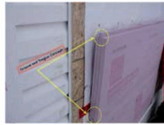
Figure 3 - Installation of VIP Panel (W3) with T&G Concept
