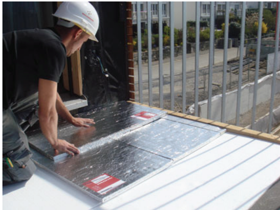
Picture 2: Roof terrace with double layer VIP. The complete insulation amounts to 24cm rock wool, 4cm VIP and 3 – 6cm foam glass.
