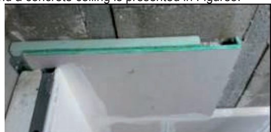
Figure 3: STB installed on-site – Thickness = 43 mm
