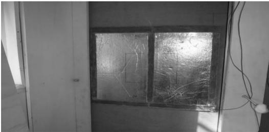
Fig. 4 VIPs assembly with structural joint
