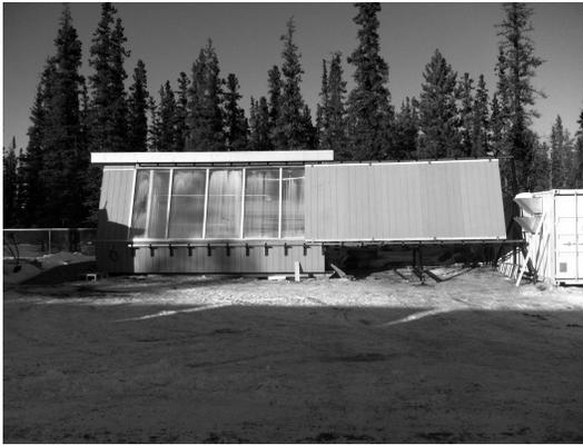
**Fig. 5 Greenhouse with VIP Sliding Door**
