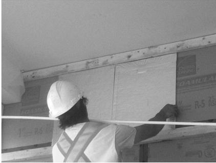
**Fig. 1 Installation of vacuum insulation panels (VIPs) at 410 Jarvis in Whitehorse, Yukon, Canada**
