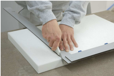
Pict.2 Cutting & tailoring simply with a knife without special tools
