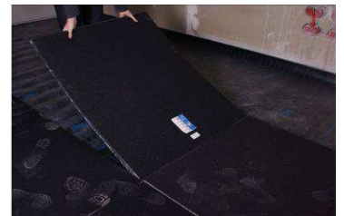
Floor insulation with Vacupor® RP-B2 on sealing membrane
