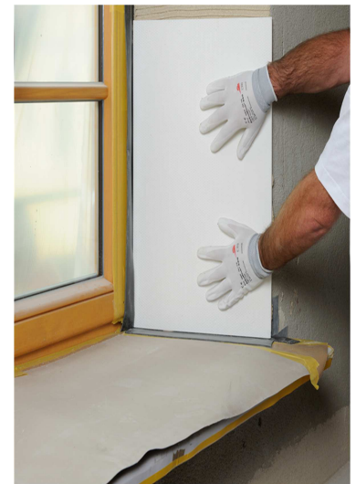
Pict.7 Window reveal using a 10 mm Sto-Aeverso board
