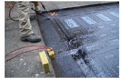
Test area 2 sealed and subsequently covered with gravel.
