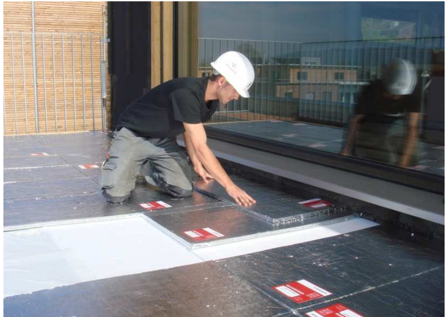
Insulation work for a flat roof terrace with double layered VIPs. Photo from SunnyWatt construction site (Source: www.vacuseed.ch/referenz )
