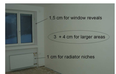
Pict.8 Example of a renovated room with StoTherm In Aeverso
