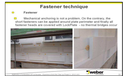
Figure 6. Mechanical fixation by fasteners
