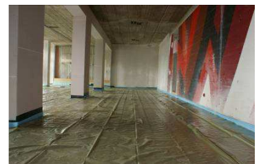
Vacupor® RP-B2 covered with flooring membrane
